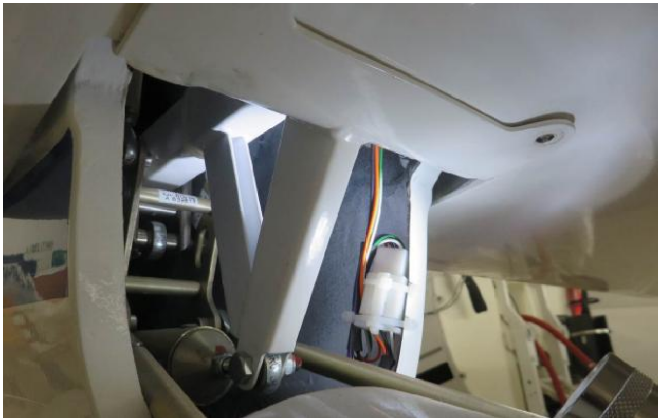
Fig. 2 – General view to area of stabilator mounting pivot to be inspected.
